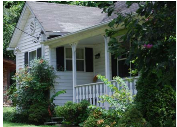
Photograph 68. Penland-Gentry House, North Elevation
