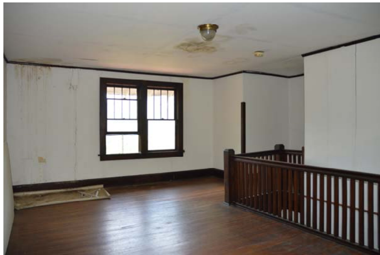
Photograph 38. William Ellerson House, Second Floor Stair Hall
