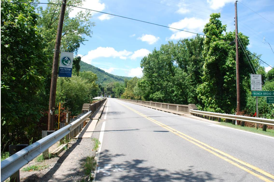
Photograph 1. Bridge No. 67, Looking West toward Hot Springs
