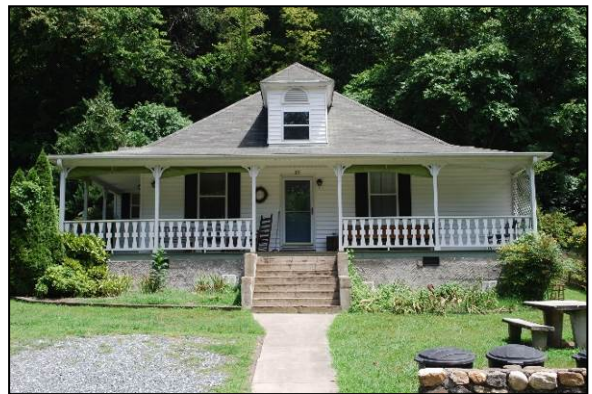
Photograph 67. Penland-Gentry House, Façade (West Elevation)
