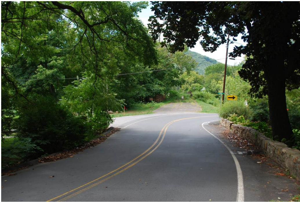
Photograph 54. Westerly View along River Road toward Old Highway Route and Former Bridge Abutment
