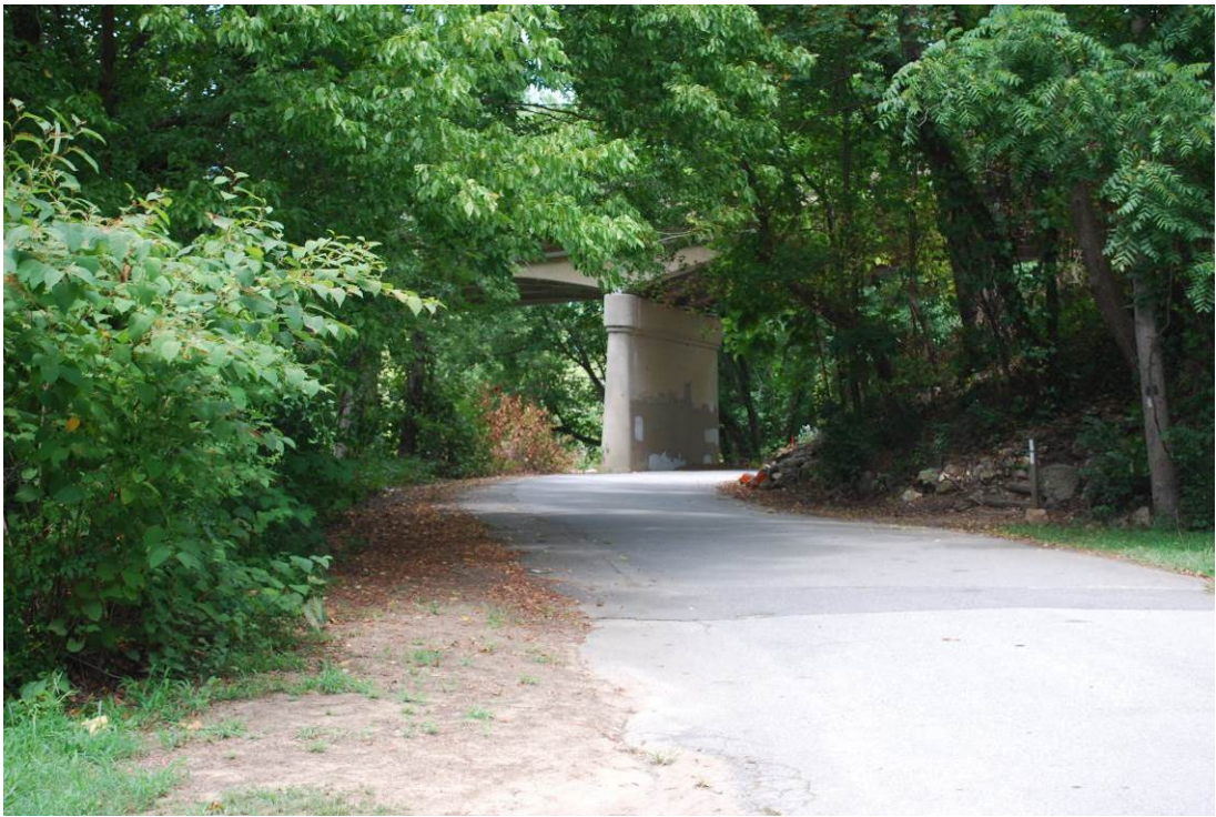
Photograph 5. Northwesterly View along Silvermine Road toward Bridge No. 67 Overhead Crossing
