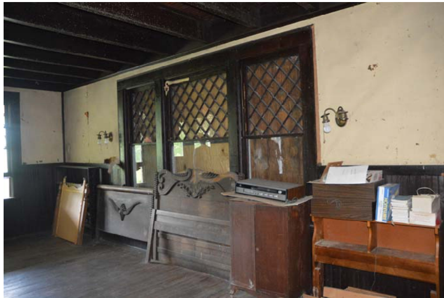
Photograph 35. First Floor Bedroom
