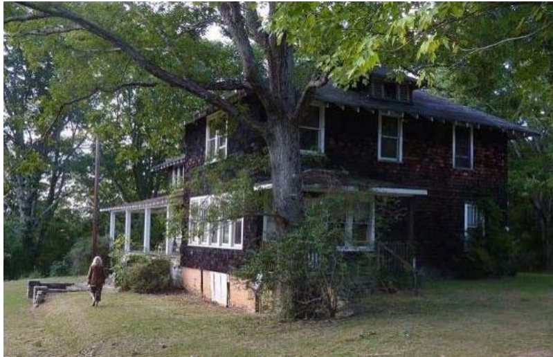
Photograph 30. William Ellerson House, Southeast Oblique
