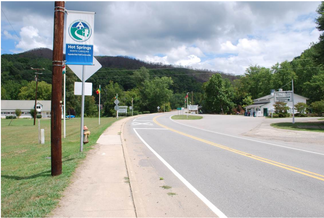
Photograph 3. Easterly View along US 25/70 toward Bridge No. 67
