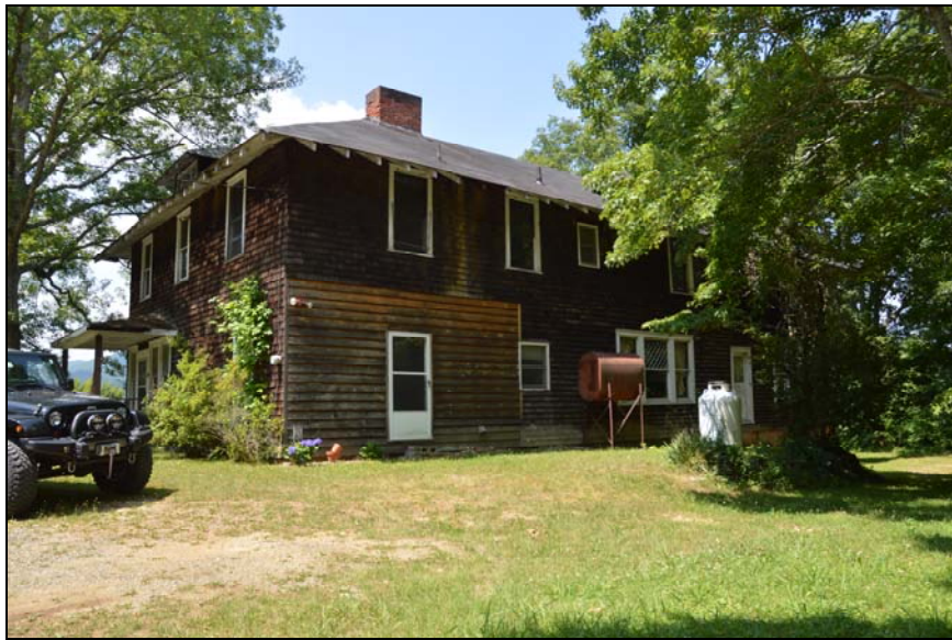
Photograph 31. Rear Elevation of the Ellerson House
