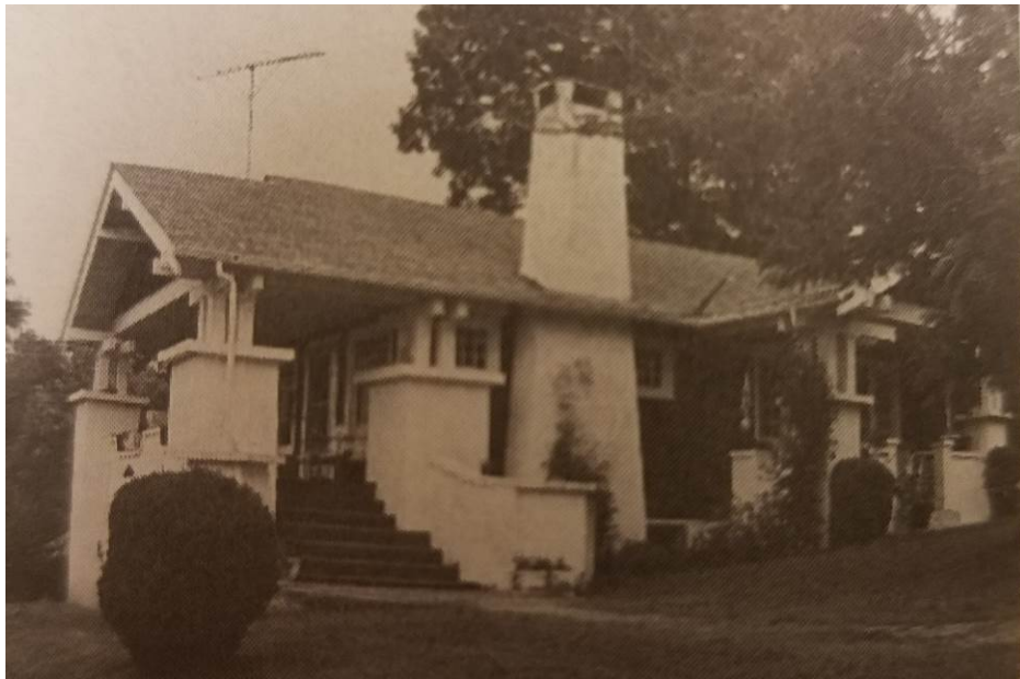
Photograph 52. Jarrett House, c.2000 Taken from: A Guide to the Historic Architecture of Western North Carolina
