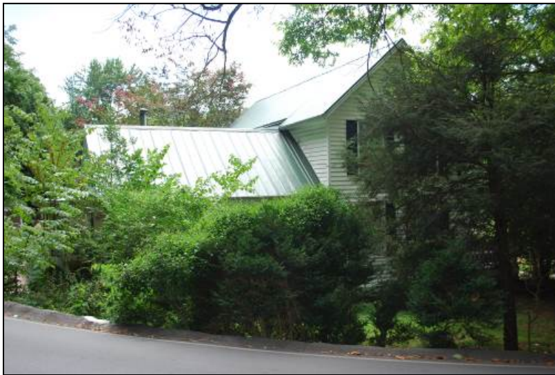
Photograph 59. J.C. Sanders House, Northeast Oblique
