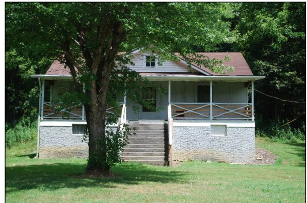
Photograph 18. J.H. Sackett House, Façade (Southwest Elevation)
