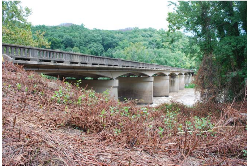
Photograph 10. Bridge No.67/Appalachian Trail
