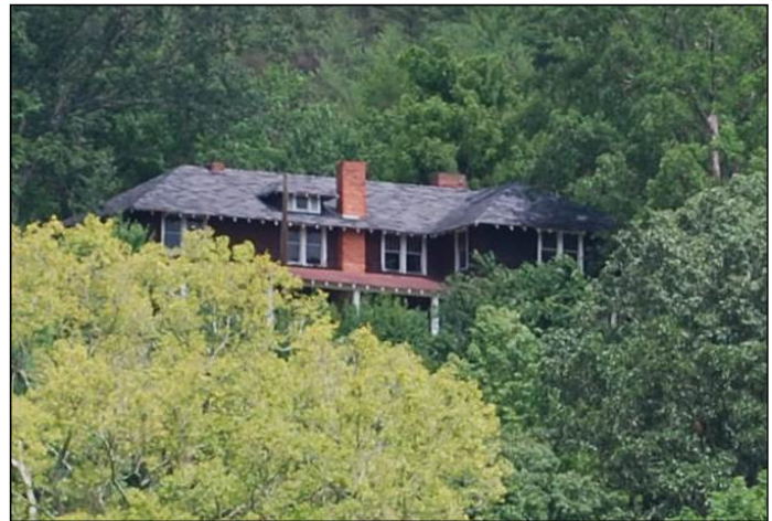
Photograph 27. William Ellerson House, Façade and Roof
