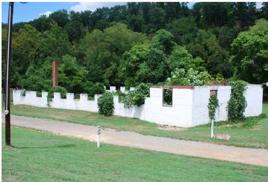
Photograph 13. Hot Springs Bath House (MD0111) Ruins (outside of APE)
